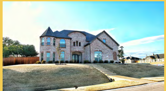
Figure 4.8 Two-story, SF home, Nolanville, TX
