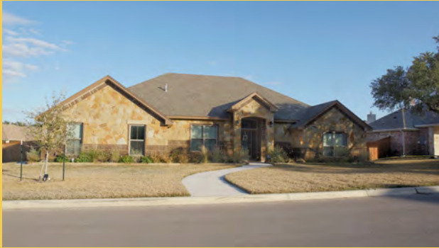
Figure 4.5 SF home, newer build, Nolanville, TX
