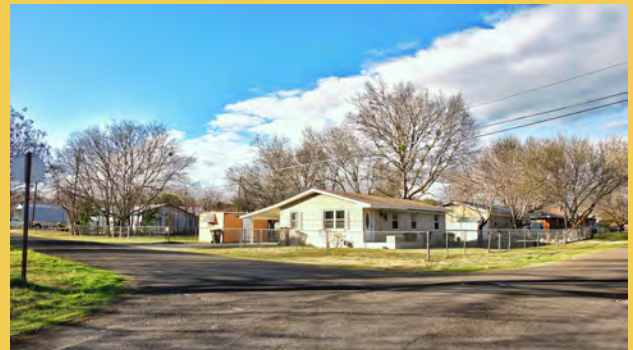
Figure 4.6 SF home, older build, Nolanville, TX
