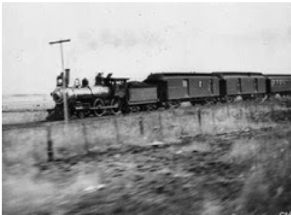
Figure 1.3 Historic photograph depicting railroad servicing Nolanville and surrounding areas.
