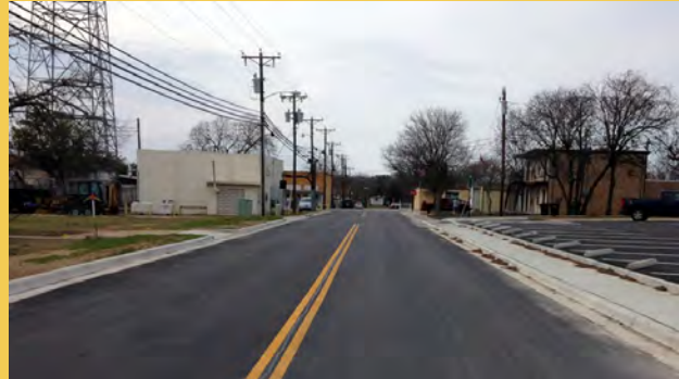
Figure 5.7 Avenue H, Nolanville, TX
